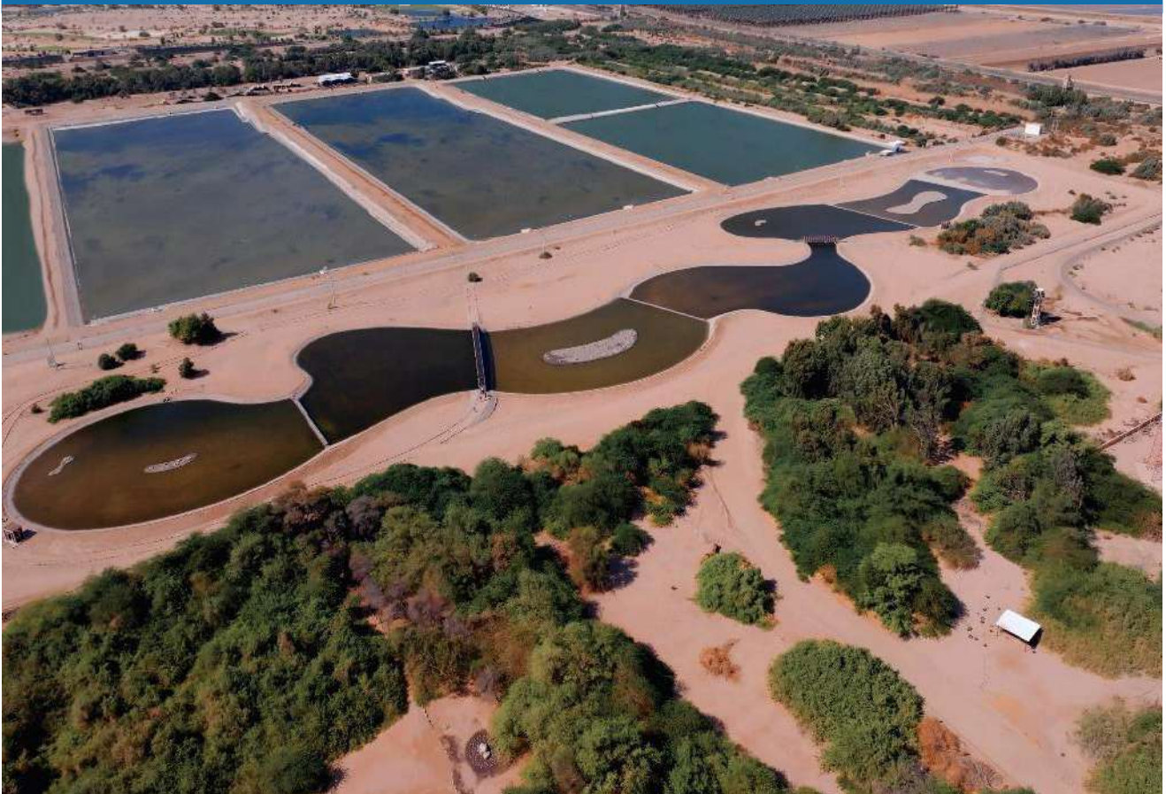
Bird Habitat at Aqaba Wastewater Treatment Plant
