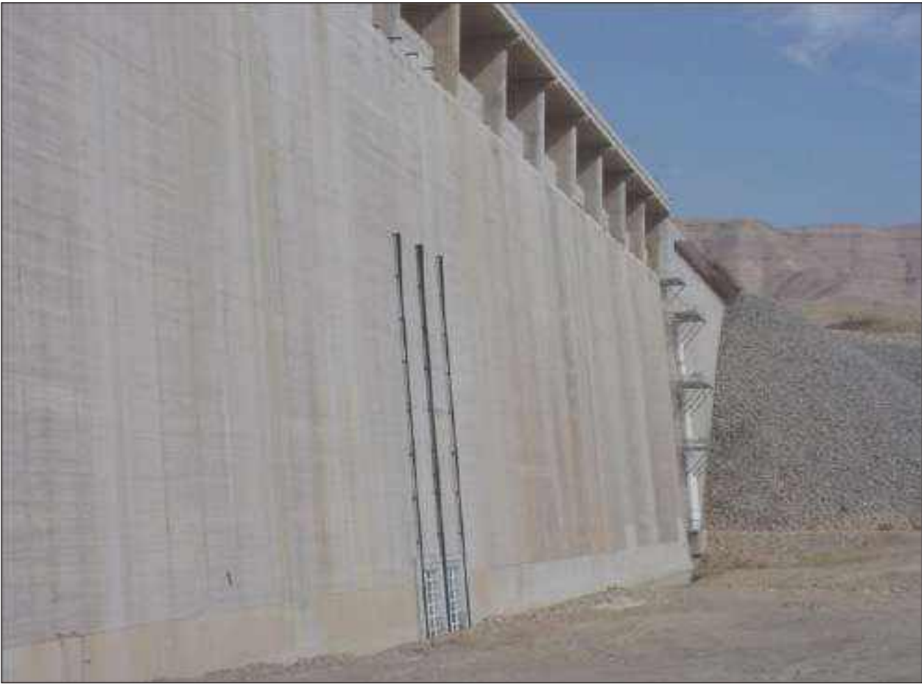
Bottom gate (sluice gate) @ 145 m asl Draw-off pipes @ 165 m asl, 175 m asl, 185 m asl
